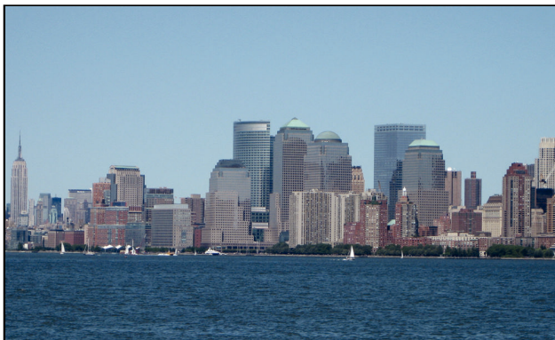
Fig. 1-4. Typical structures covered by NFPA 70E
