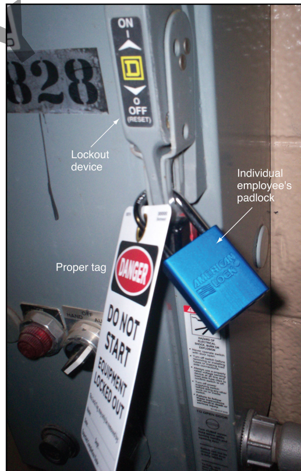
Fig. 1-2. Lockout/tagout application
