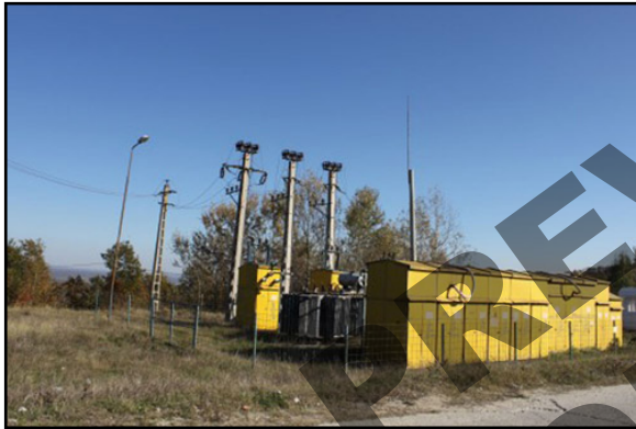
Fig. 1-6. Electrical unit substation
