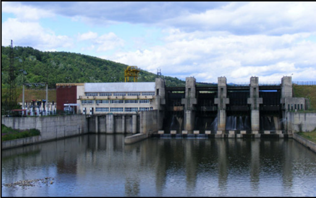
Fig. 1-5. Hydropower electrical generation plant
