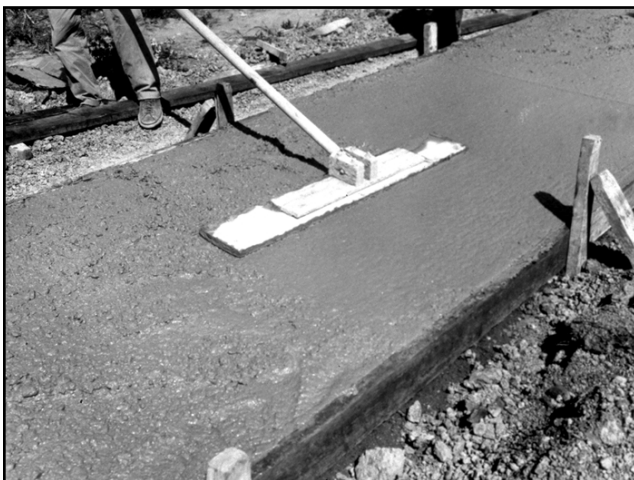
Fig. 1-9. Floating concrete with a bull float
