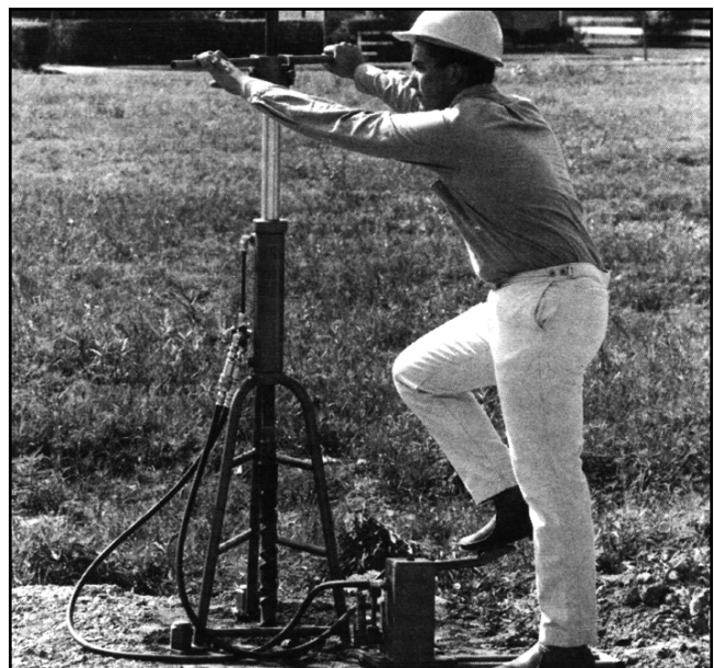
Fig. 1-1. An engineer drilling for a soil sample
