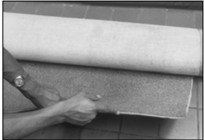
Fig. 1-2. Carpet edges are not bound
