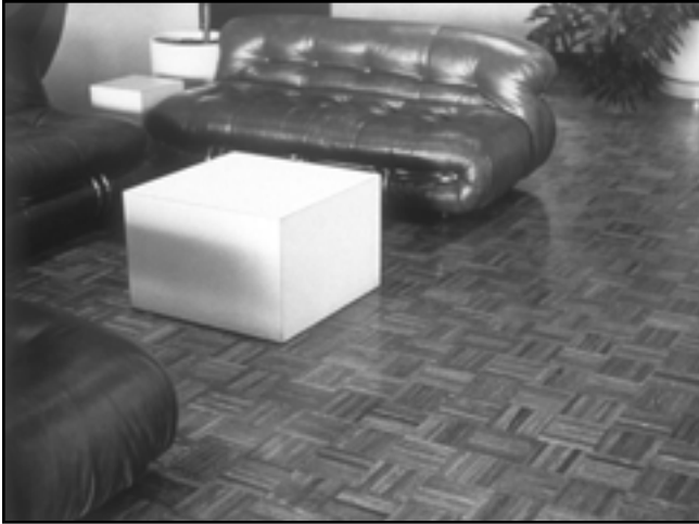
Fig. 1-11. Parquet floor in office lobby
