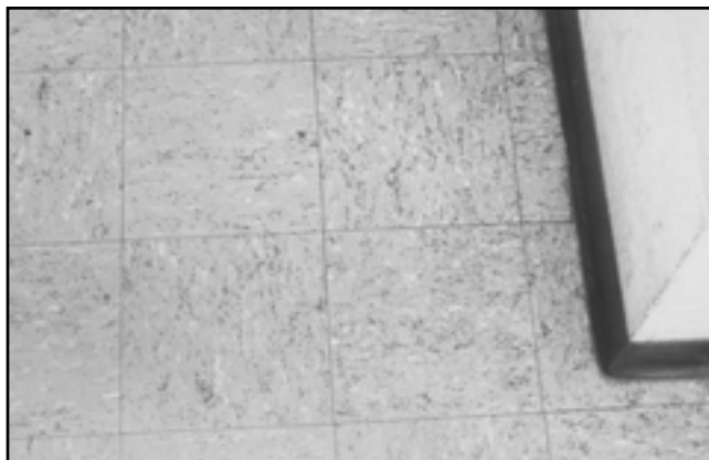
Fig. 1-1. Vinyl composition tile floor in hallway
