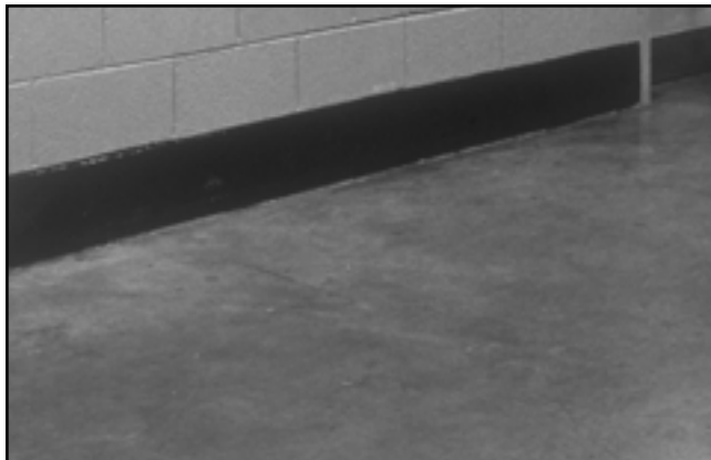
Fig. 1-3. Concrete floor surface
