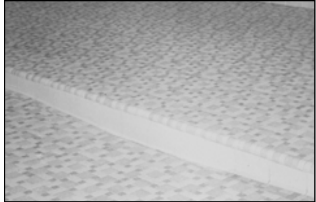
Fig. 1-6. Ceramic tile flooring in locker room
