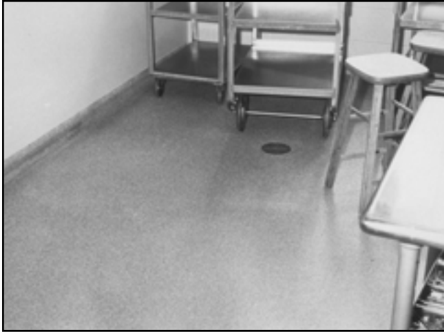
Fig. 1-9. Epoxy floor in cafeteria
