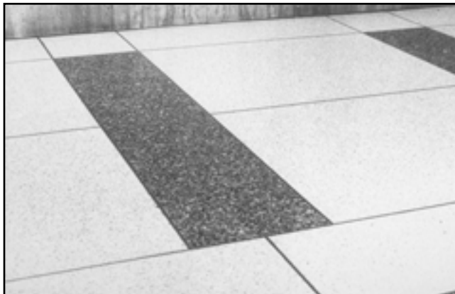
Fig. 1-4. Terrazzo panels separated by strips
