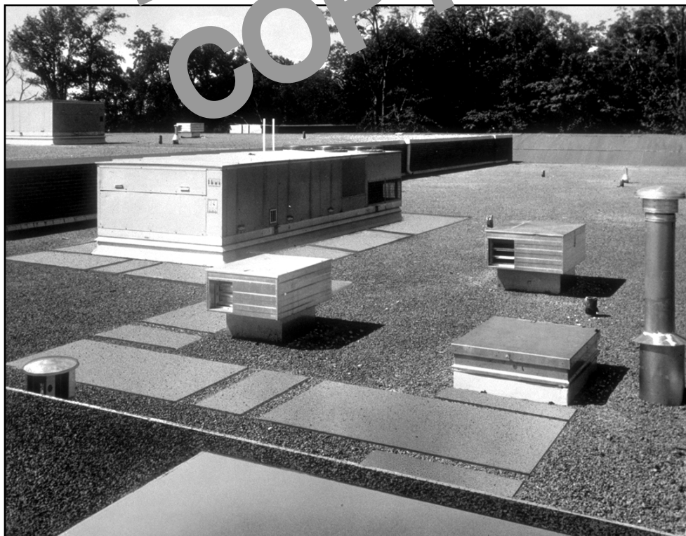
Fig. 1-7. Service walkway made of heavy felt pads
