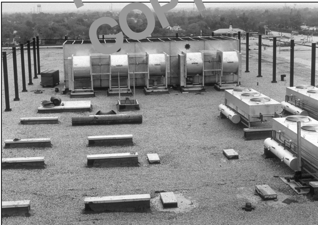
Fig. 1-2. Common type of built-up flat roof
