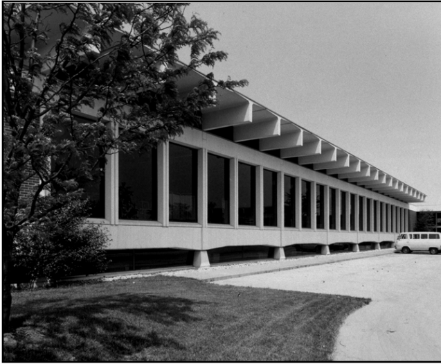
Fig. 1-4. A modern roof of precast concrete
