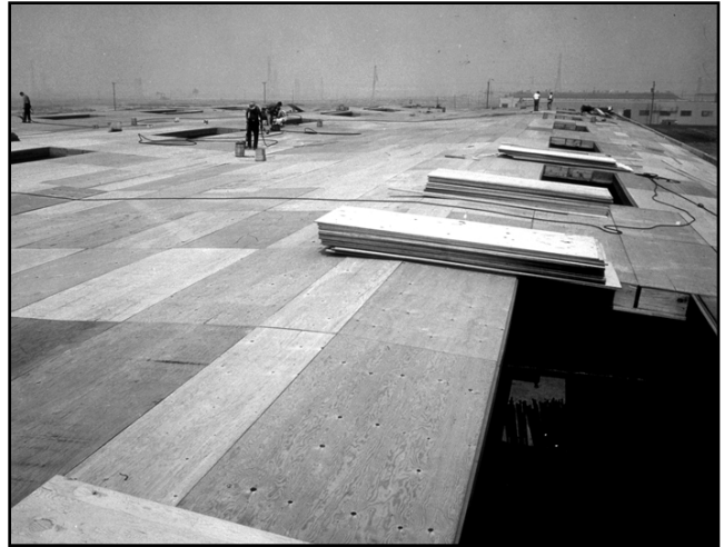
Fig. 1-3. A plywood deck before building up
