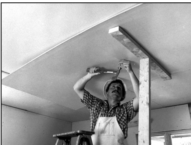
Fig. 1-11. Support ceiling panels while securing them
