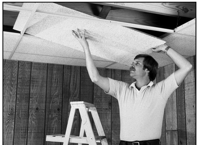
Fig. 1-14. Installing a suspended tile ceiling
