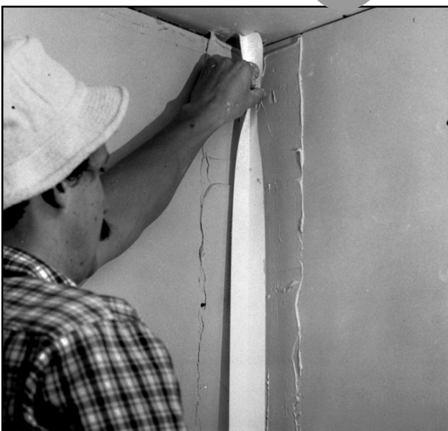
Fig. 1-7. Applying tape in the corner of a room
