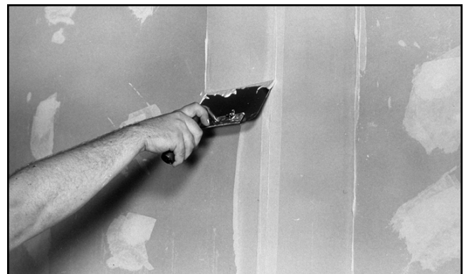
Fig. 1-1. Applying tape and cement to wall seam
