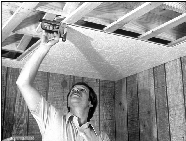
Fig. 1-13. Stapling ceiling tiles to furring strips
