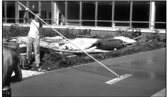
Fig. 1-16. Levelling a concrete slab with a float
