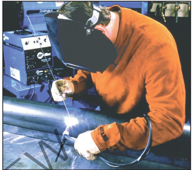
Fig. 1-15. Welding steel pipe
